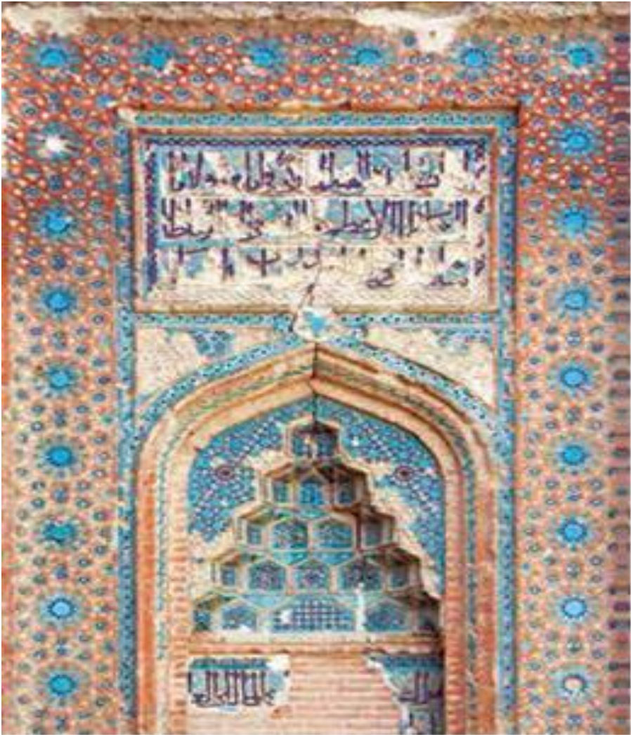
Fig. 11 Brick working of glazed tiles in Gonbad-e-Ghaffariyeh
