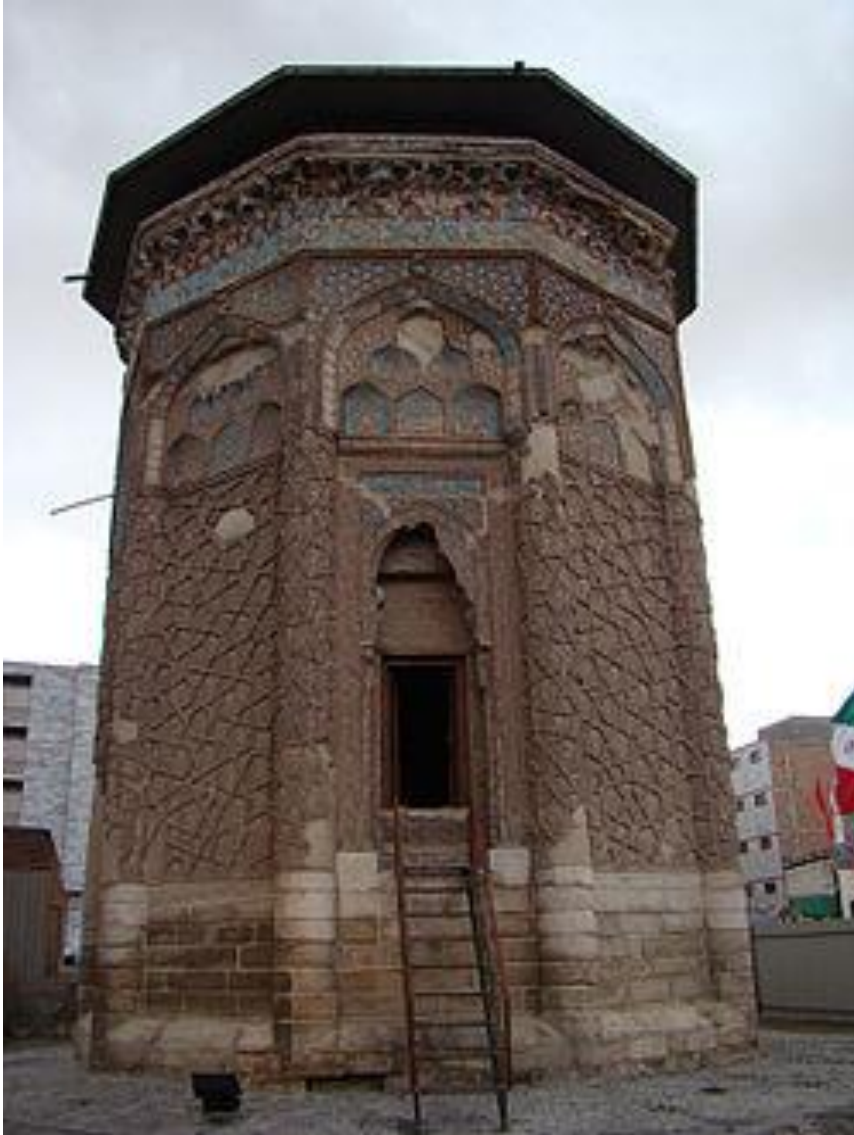
Fig. 1 General view of Gonbad-e-Kabood
