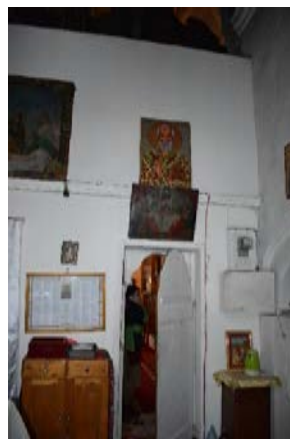
Fig. 35. False wall behind the iconostasis
