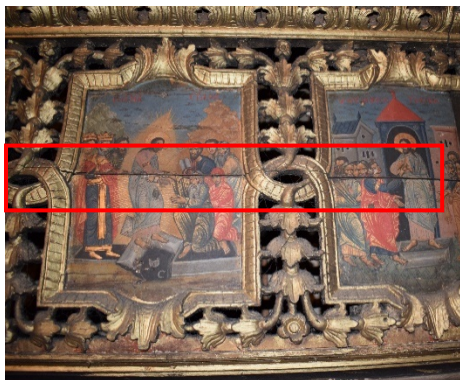
Fig. 36. Fractures on the wood merge
