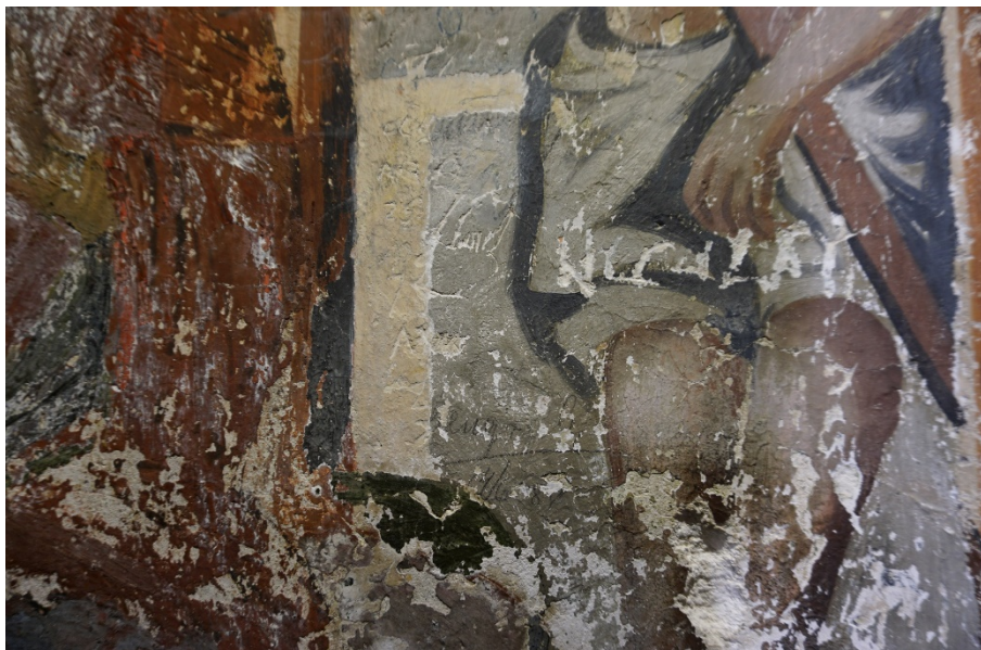
Fig. 20. Sucevița Monastery, exonarthex, detail during work.
