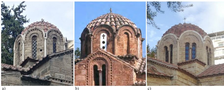
Fig. 5. Completion of the dome drums with a continuous row of arched gables: a) Athens. Kapnikarea, b) Plataniti. Church of Metamorphosis, c) Athens. Hagioi Theodoroi.
